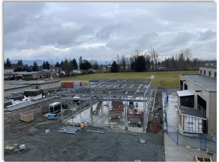
Structural framing of shops
