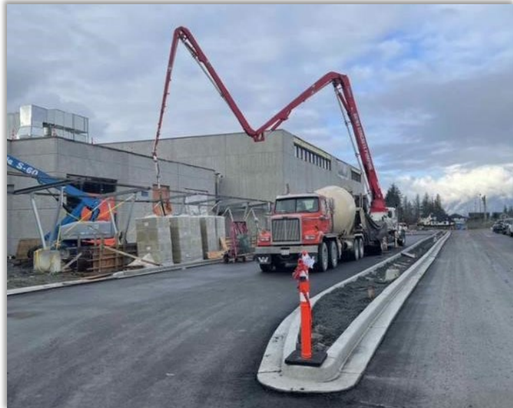
Curbing and Paving of parking lot entrance
