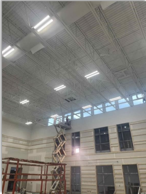
Drywall installed in main hallway
