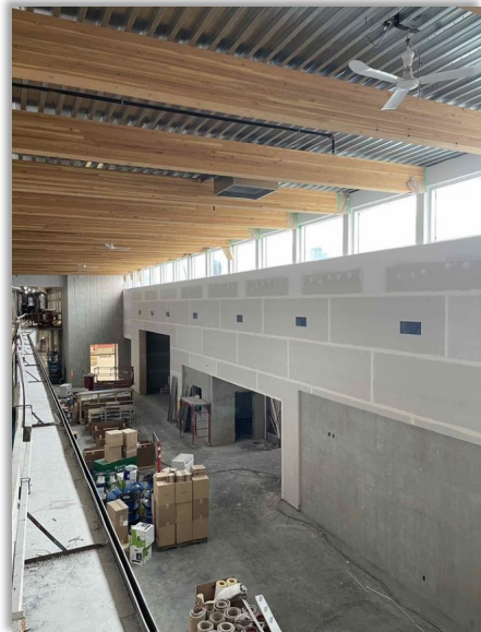
Drywall installed in main hallway
