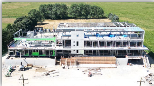
* New East Side Elementary Construction
